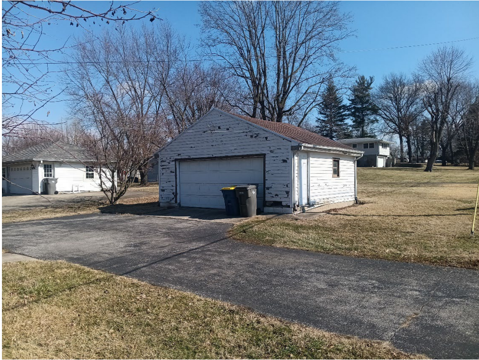
Exhibit 7: The garage that is currently on the subject site looking northeast.
