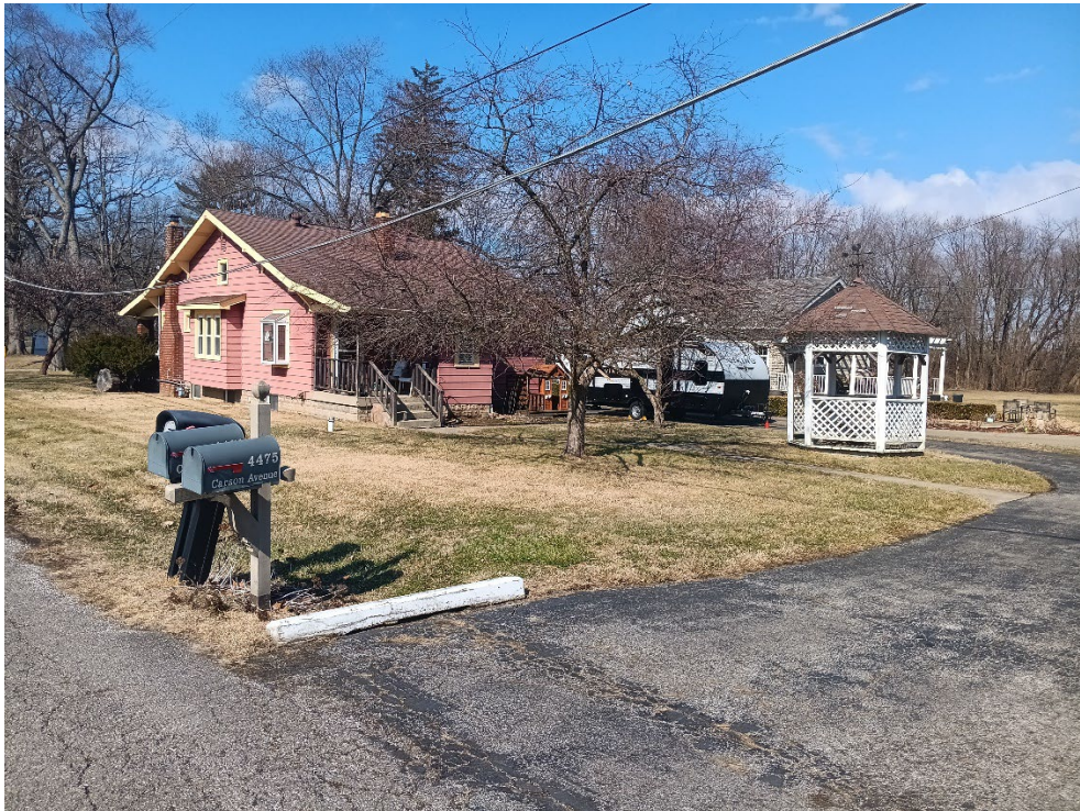
Exhibit 6: The back of the primary structure on the subject site.
