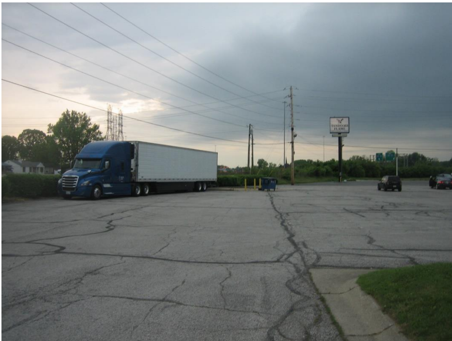
Photo of approximate area for the requested one and one-half drive-through stacking spaces in the front yard, looking south.
