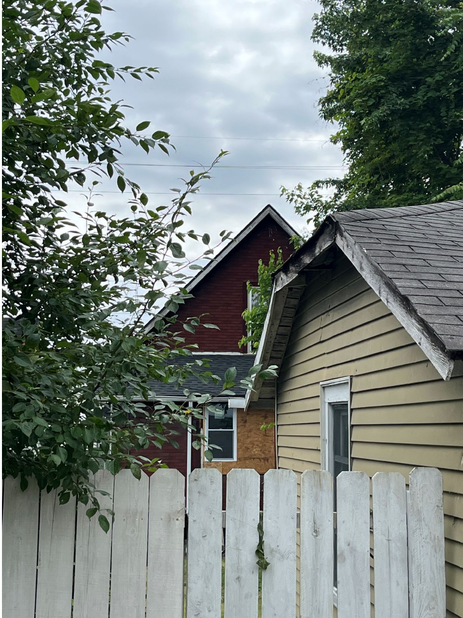
Photo 8: 2422 Prospect Street as seen from the alley
