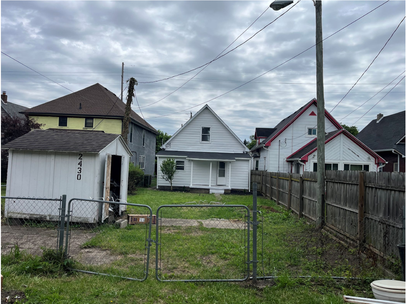
Photo 8: 2430 Prospect Street as seen from the alley
