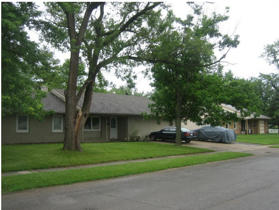
Adjacent dwellings to the southeast.
