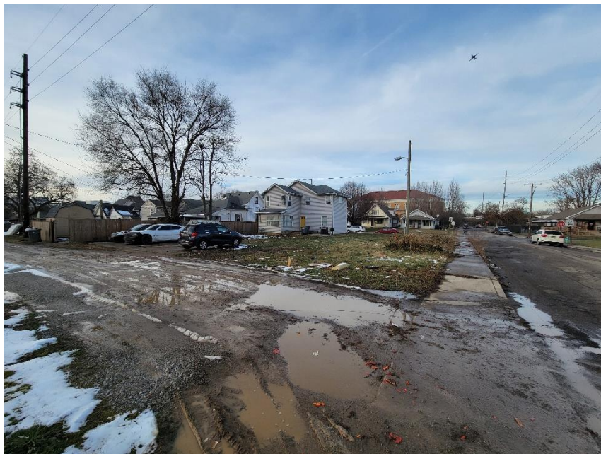
Photo 2: Subject Site Viewed from Southeast
