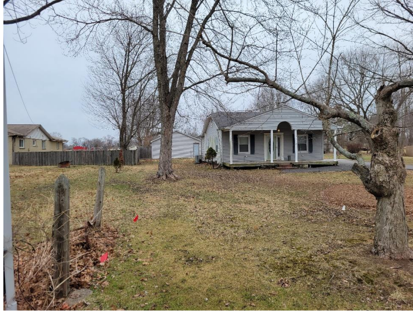
Photo 1: Existing Residence and Detached Structure Viewed from Stanley
