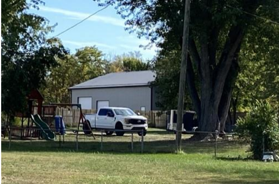
Photo 3: Newer Detached Structure Viewed from Northwest (October 2025)
