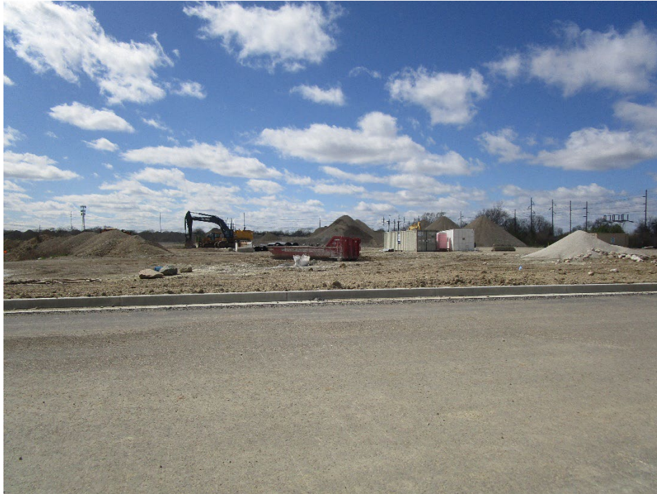
View of site looking west across Fintail Drive
