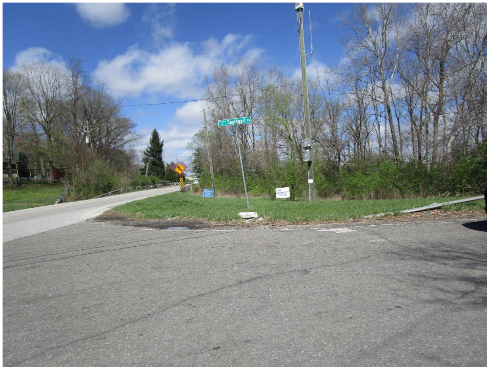
View looking north across intersection of South Mooresville Road and West Southport Road
