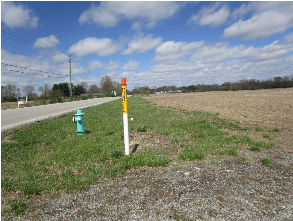
View looking east along West Southport Road
