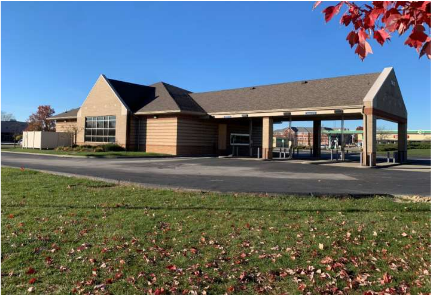
Photo of the existing east building façade.
