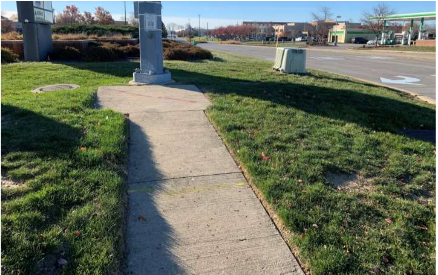
Photo of the end of the sidewalk along Northwest Boulevard.
