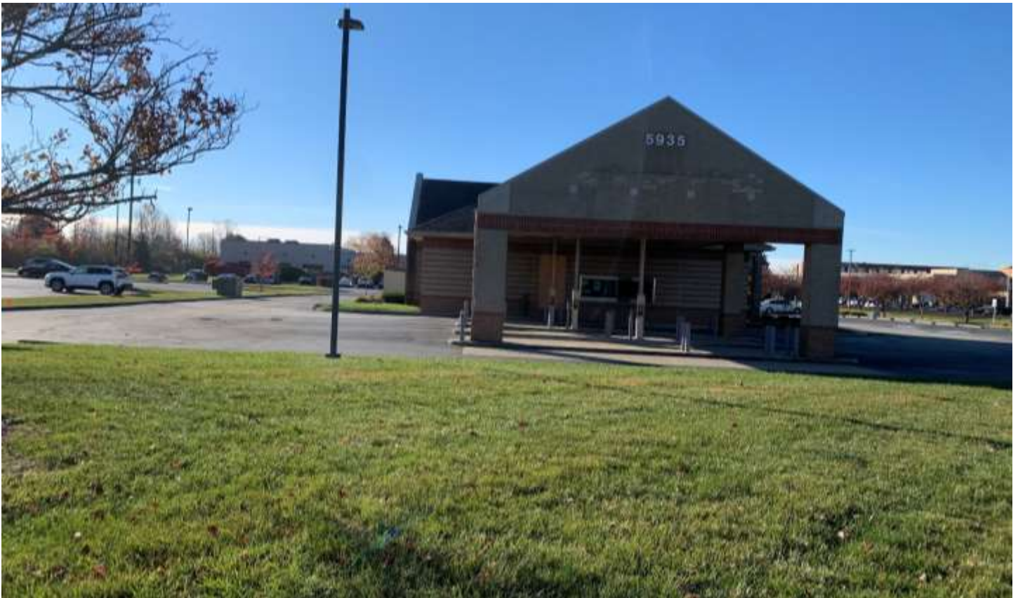
Photo of the existing north building façade.
