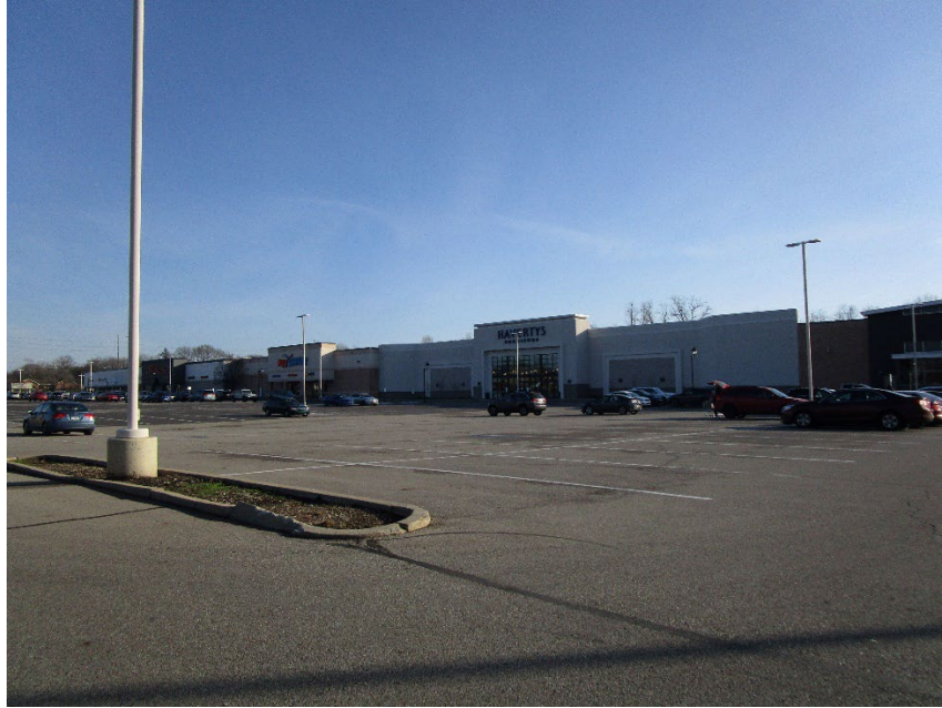
View of site looking southeast
