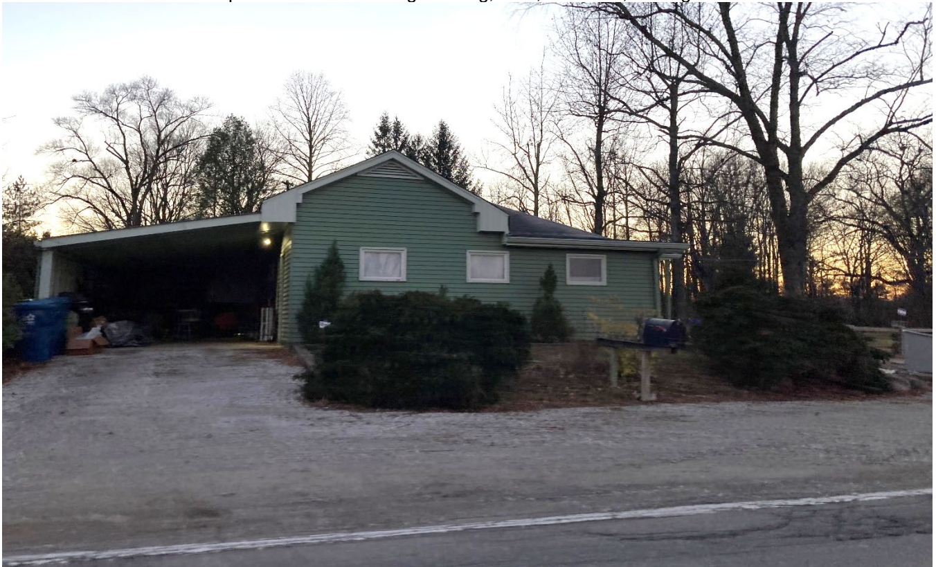
Existing dwelling viewed from Southeastern Avenue, looking west
