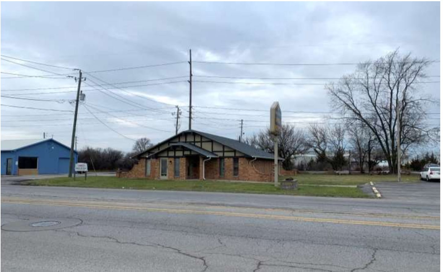
Photo of the Subject Property: 8550 East 30th Street
