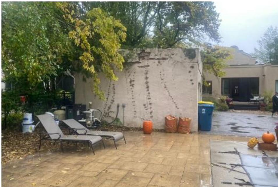
Photo 4: Western Elevation of Existing Garage (taken October 2023)
