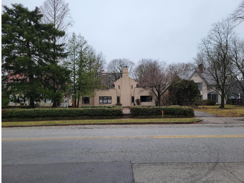
Photo 1: Existing Residence Viewed from Across Pennsylvania (East)
