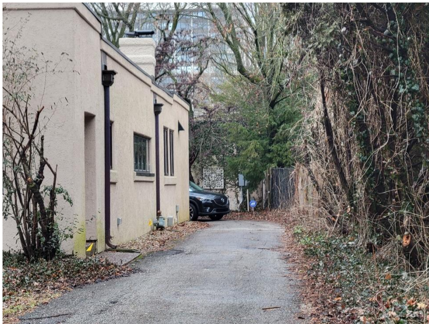
Photo 2: Existing Garage Viewed from ROW to East (Partially Obstructed View)
