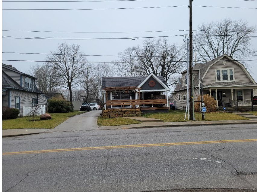
Photo 1: Existing Restaurant Viewed from Across Thompson (Northeast)
