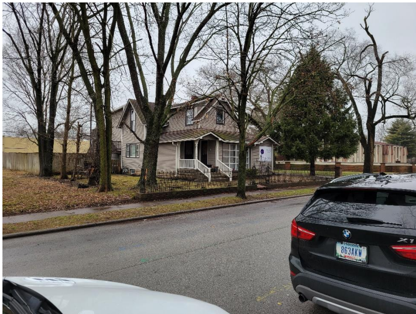
Photo 4: Adjacent Property to the Northwest
