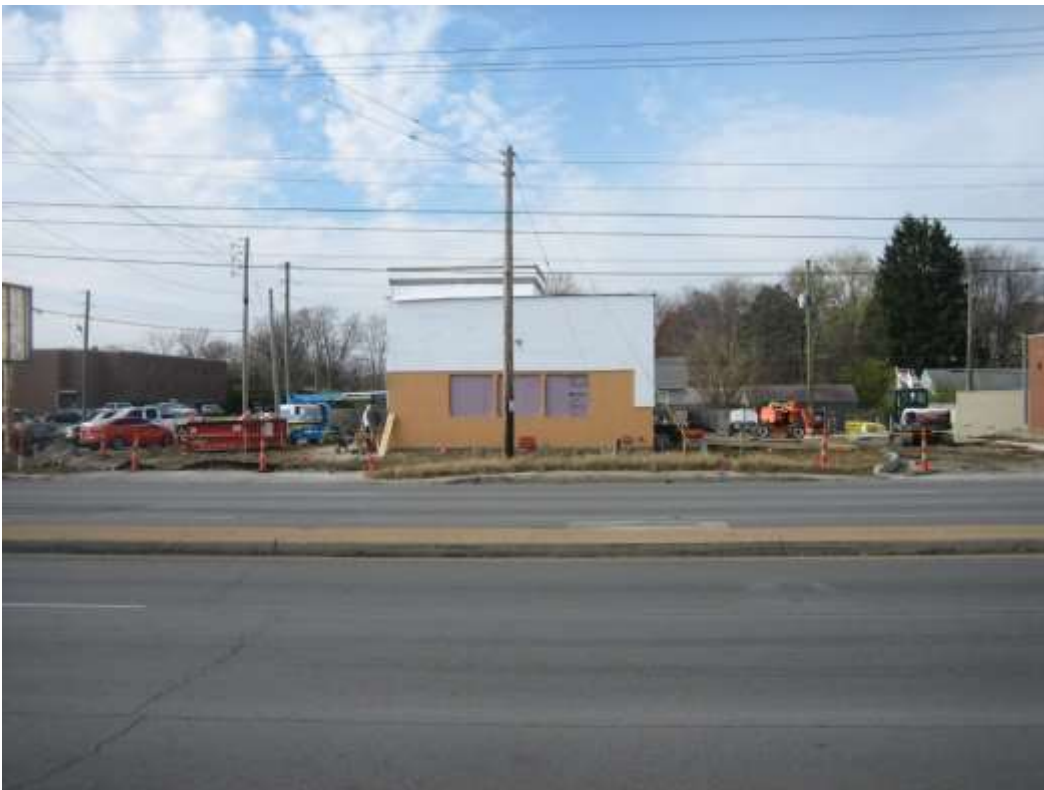
View of subject site, proposed building under construction, looking west from North Keystone Avenue.
