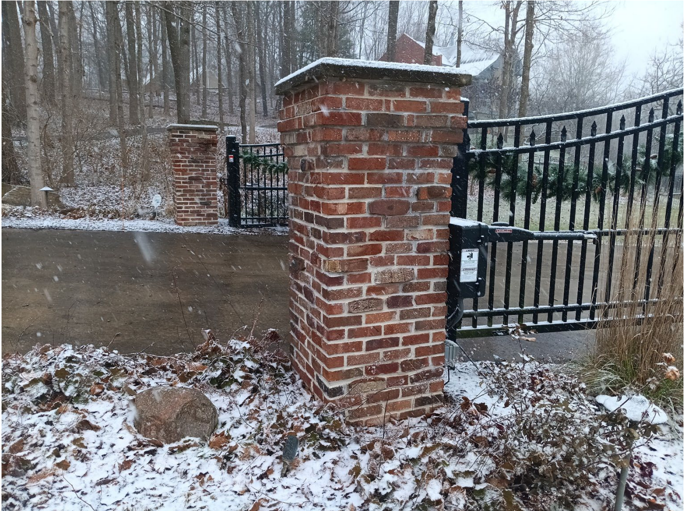
Exhibit 7: West Driveway Entrance, the bricks of the fence will match the bricks of these columns.
