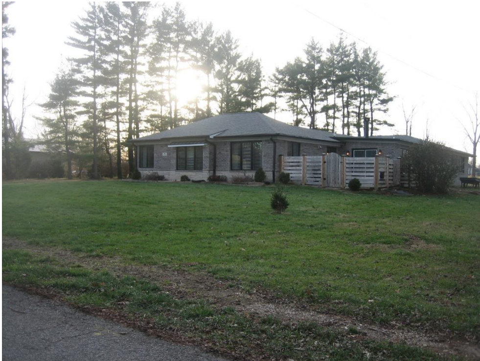
Photo 6 - Adjacent property to the west that is zoning complaint.
