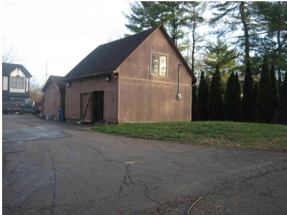
Photo 2 - Subject property existing garage to be removed and replaced with a larger garage, looking southeast.
