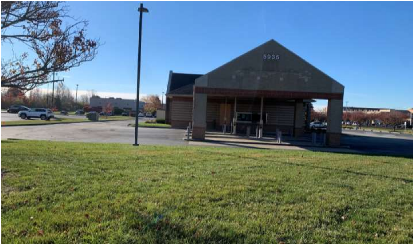
Photo of the existing north building façade.
