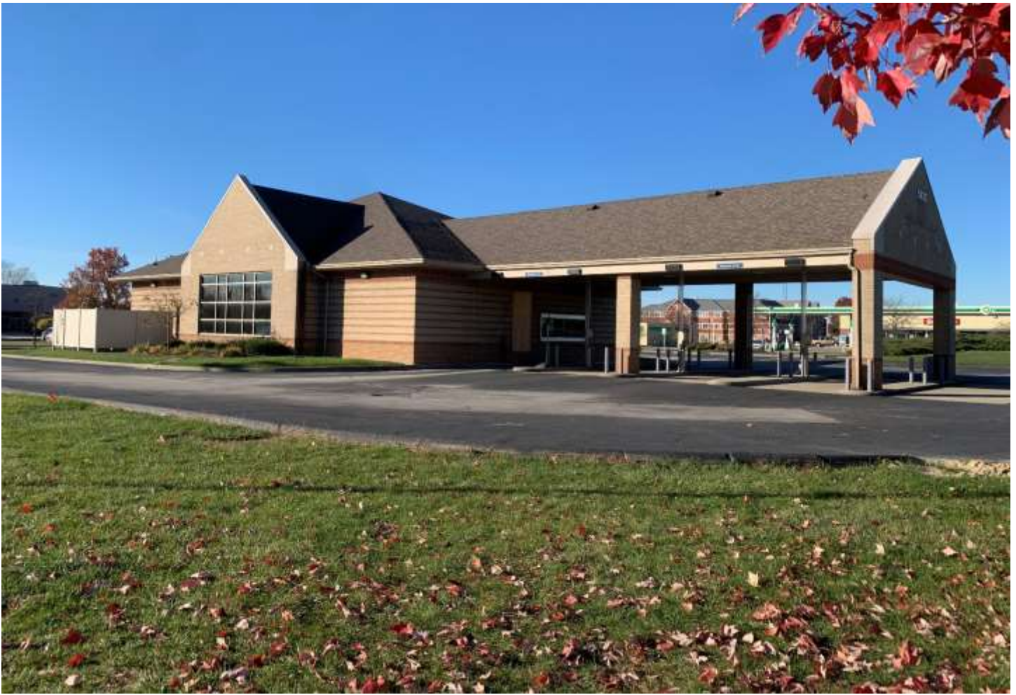
Photo of the existing east building façade.
