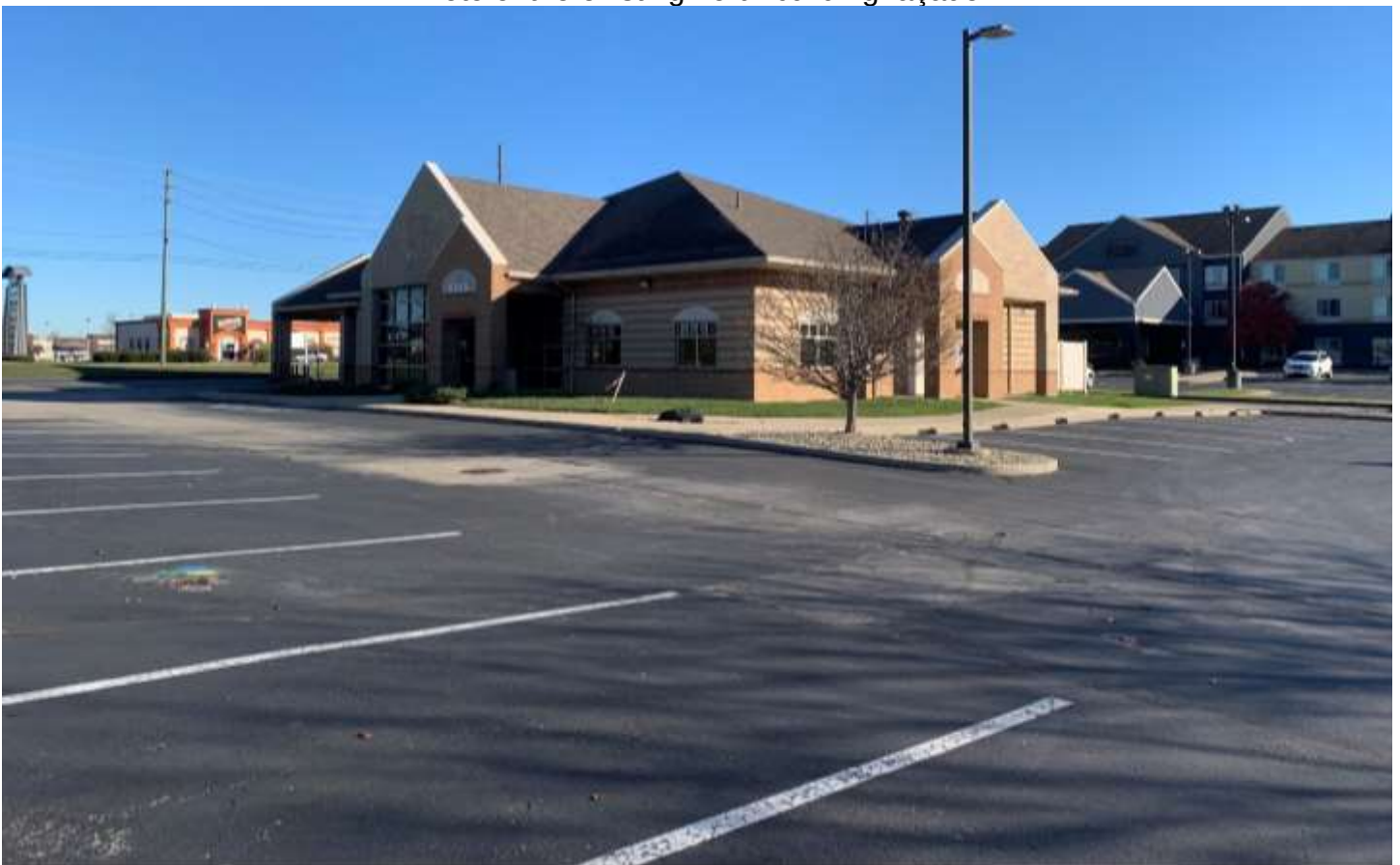
Photo of the existing west building façade.
