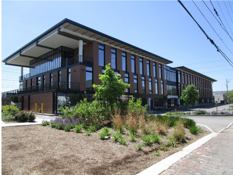
View looking southwest at adjacent building to the west
