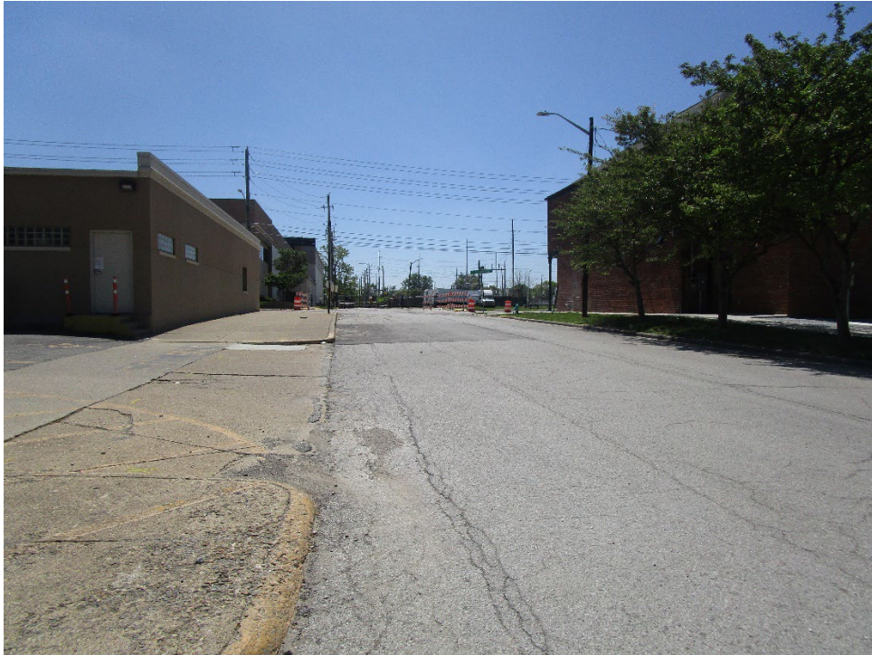
View looking south along North Arsenal Avenue
