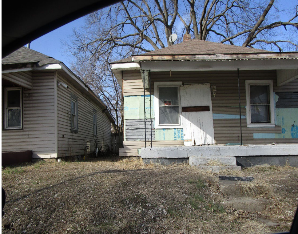
View of site looking north across Astor Street
