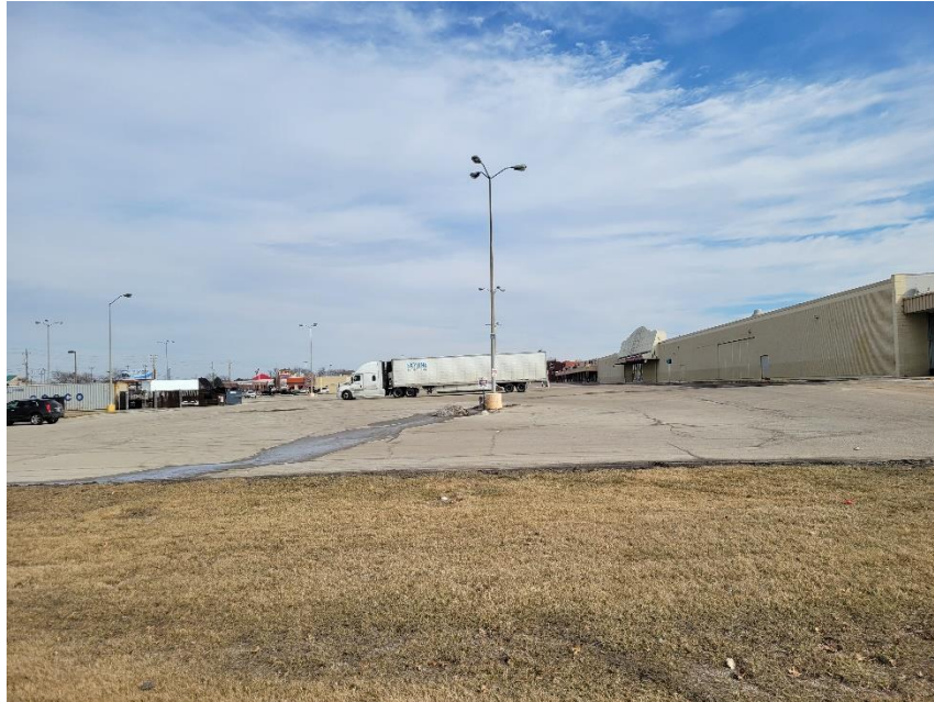
Photo 5: View from East along Emerson
