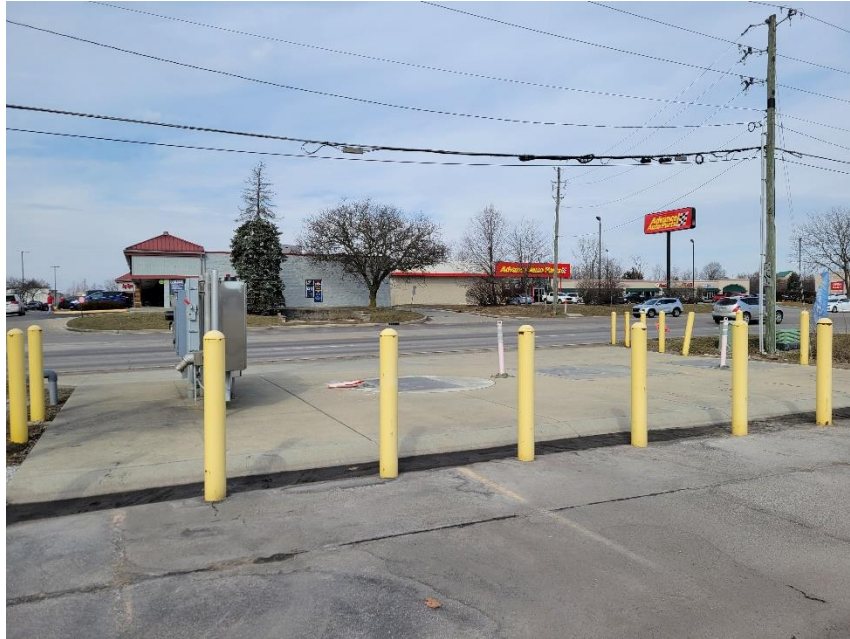
Photo 7: Existing Utility Site along Southern Side of Thompson
