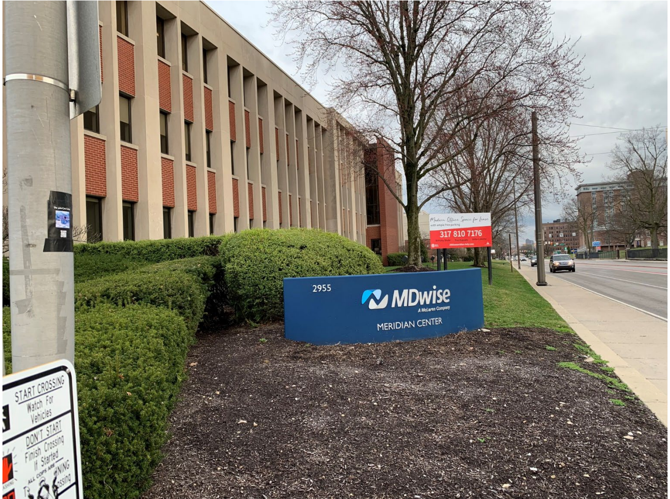
View of site along Meridian Street
