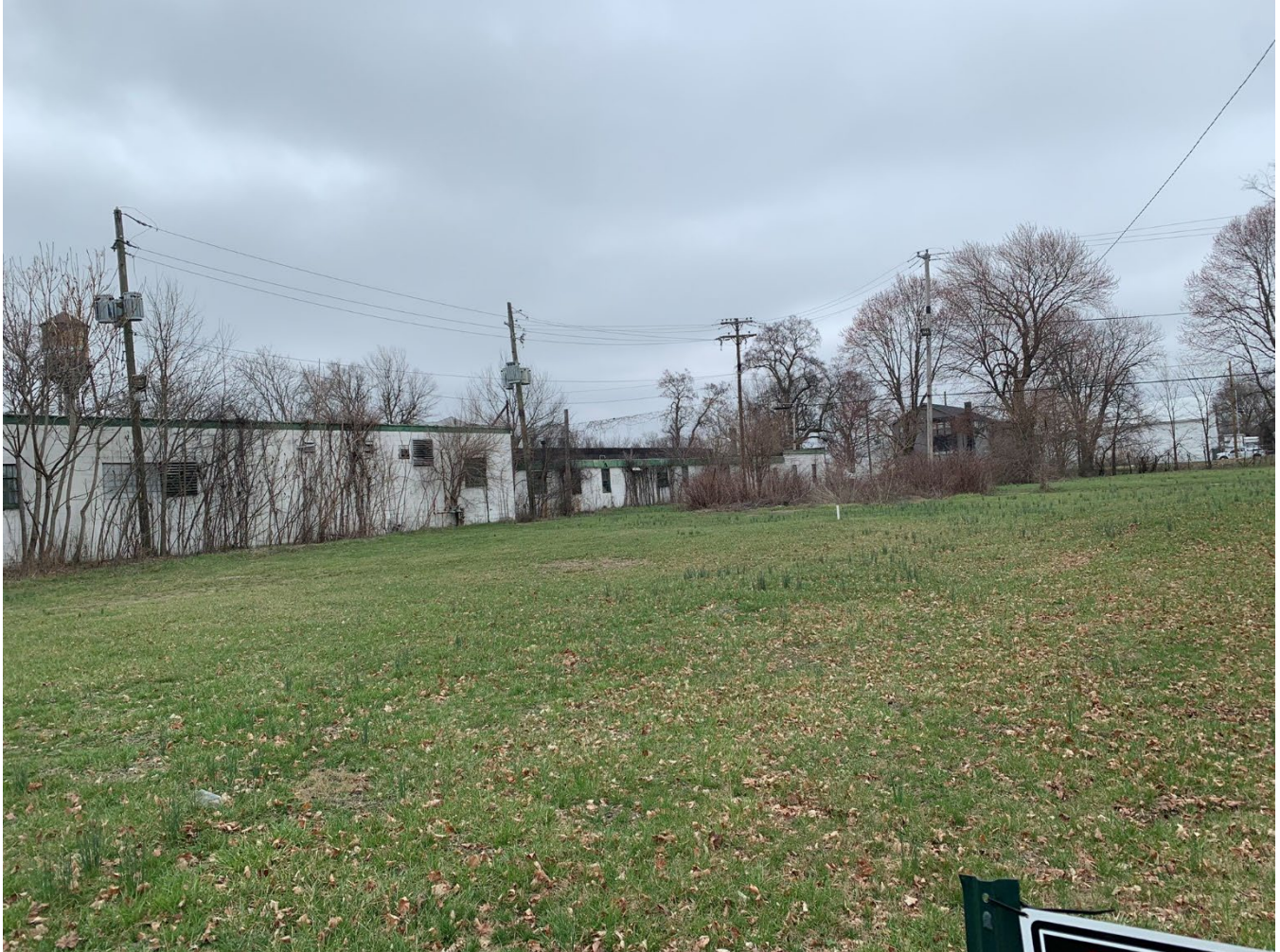
View of a large portion of the subject site
