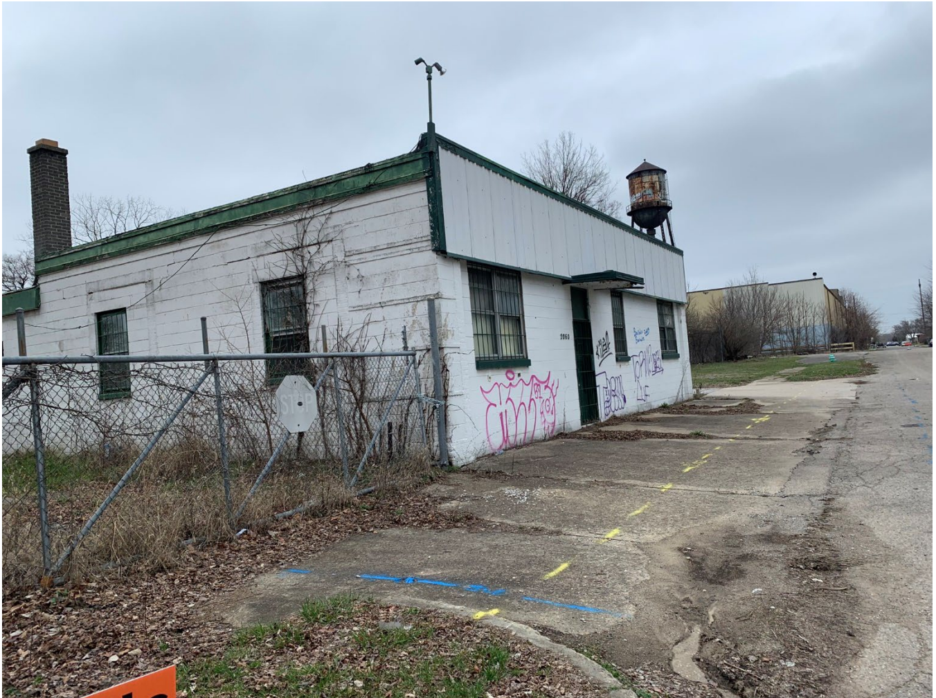
View of an existing industrial building along the northern portion of the site, from Yandes Street
