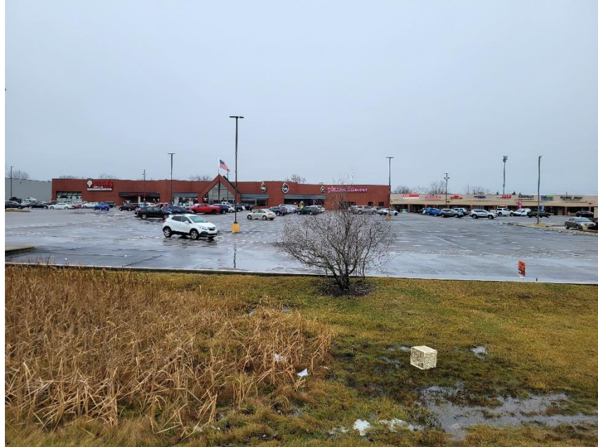
Photo 1: View from North along Thompson
