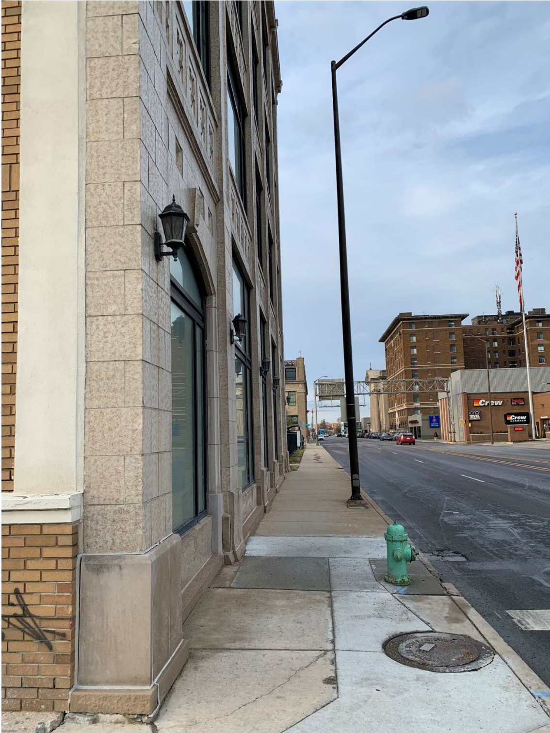
View along Meridian Street looking north
