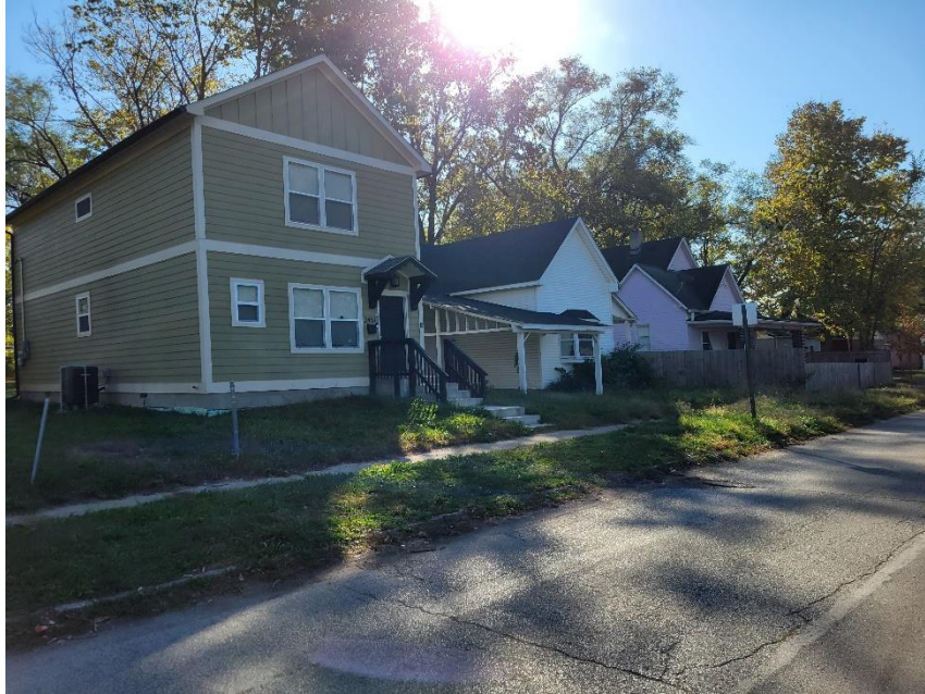
Photo 5: Adjacent Property to South
