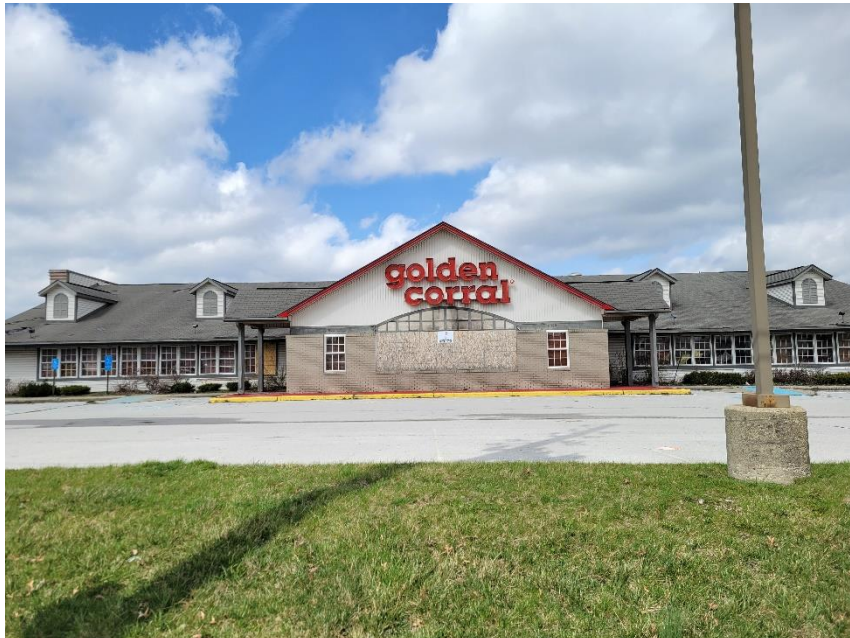
Photo 2: Property Currently Occupying Block A
