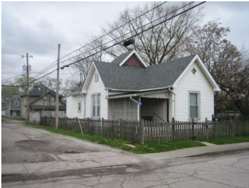
Adjacent single family dwelling to the north, looking west.
