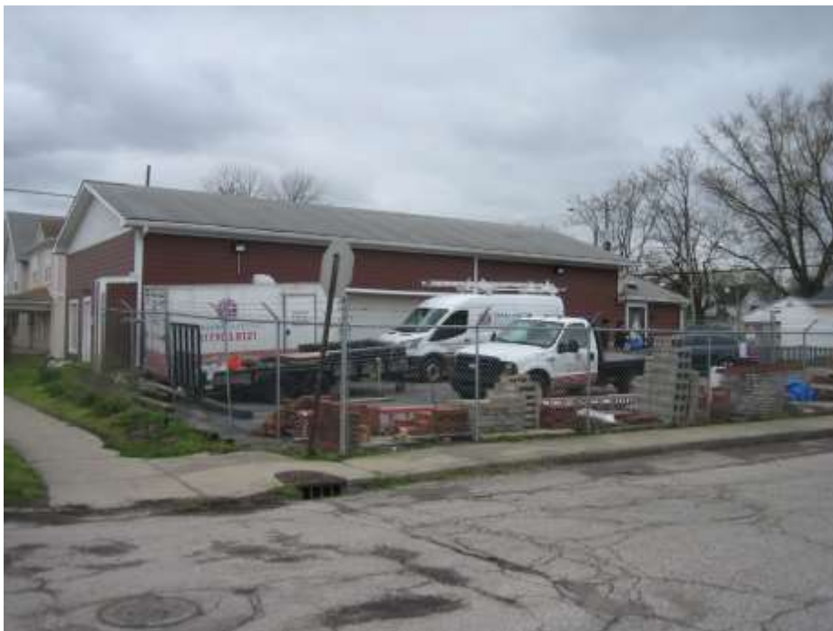
Subject site side yard with existing fencing, looking northwest.
