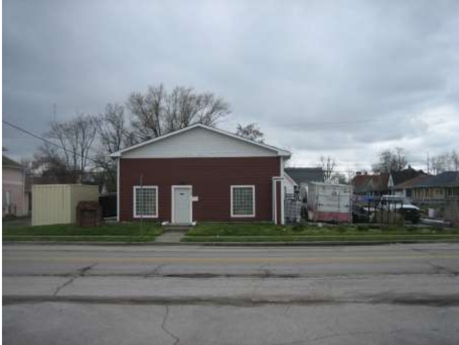
Subject site, looking north
