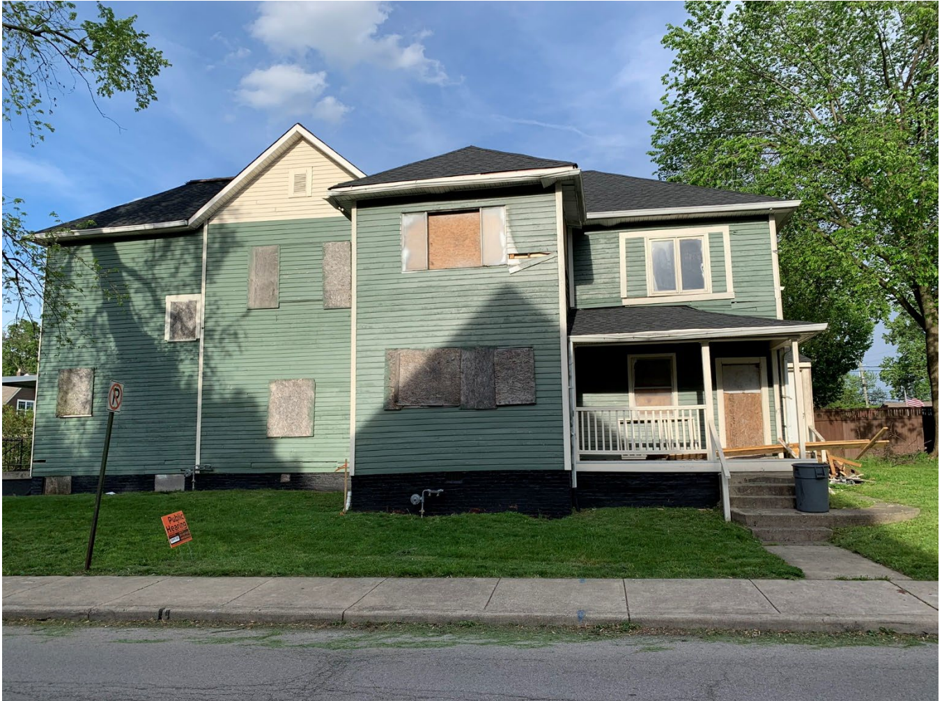
View of existing dwelling along Laurel Street
