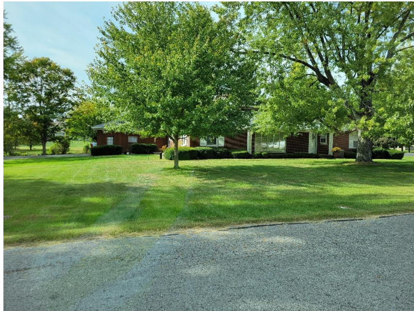
Photo 1: Existing 4344 Wanamaker Residence Viewed from East
