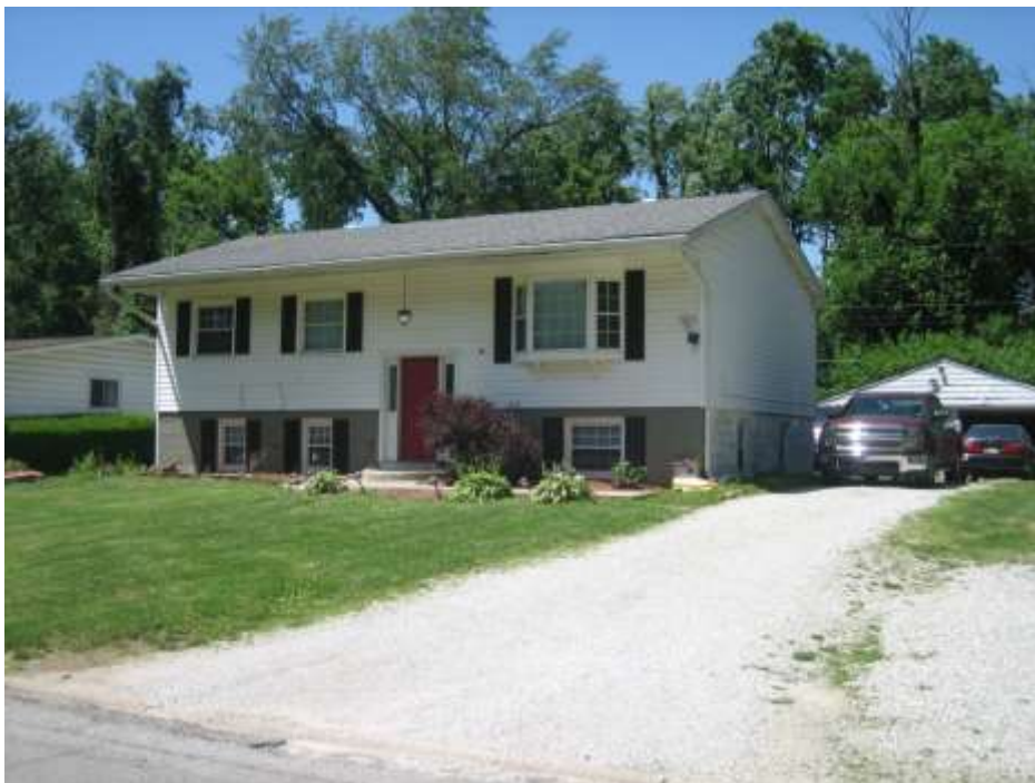
Photo of adjacent single-family dwelling to the west, looking north.
