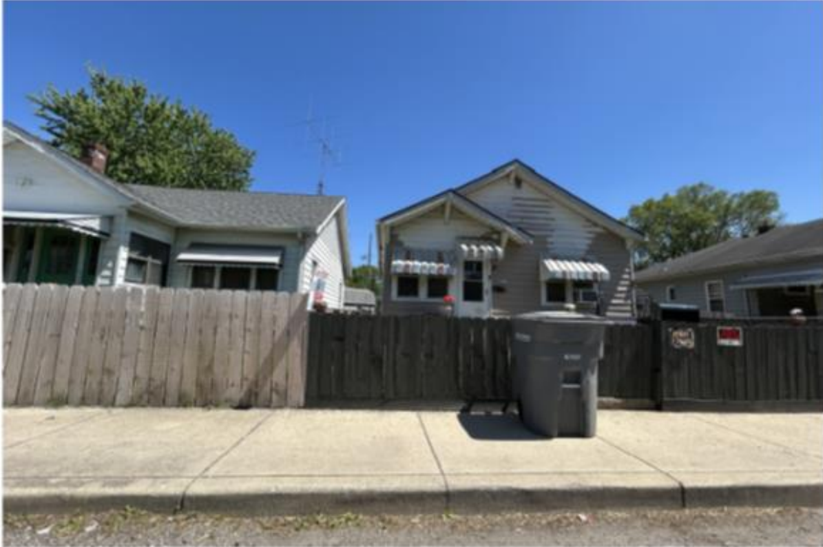
Photo 1: A BNS inspector's photo of the front of the front of the property.
