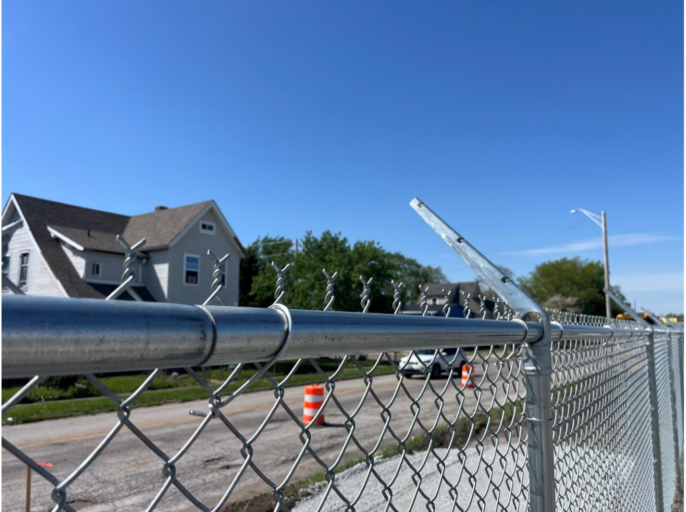
Photo 2: Close up of fence showing where barbed wire will be installed
