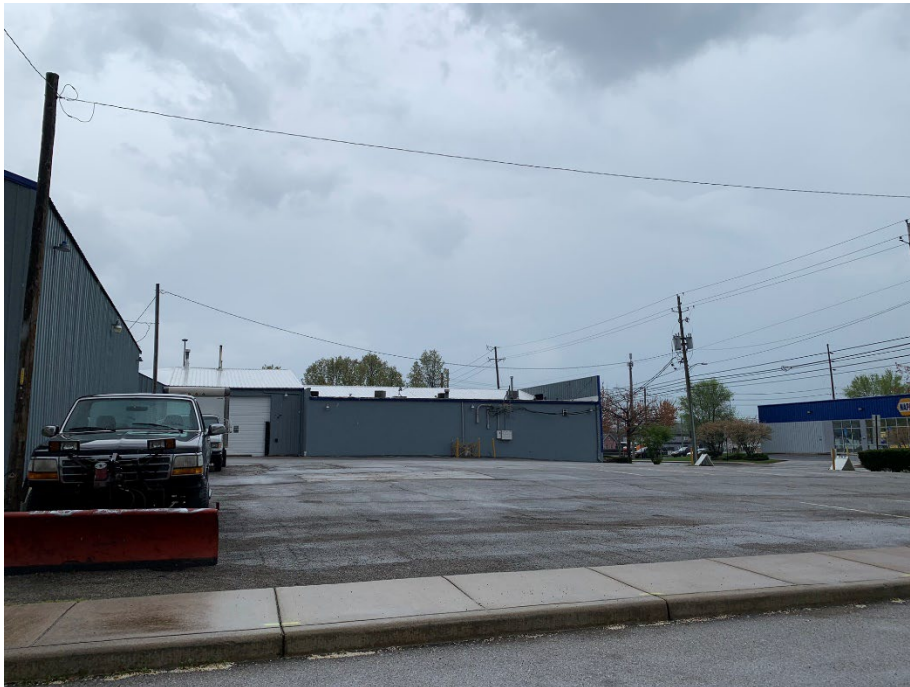
Views of existing buildings on the site
