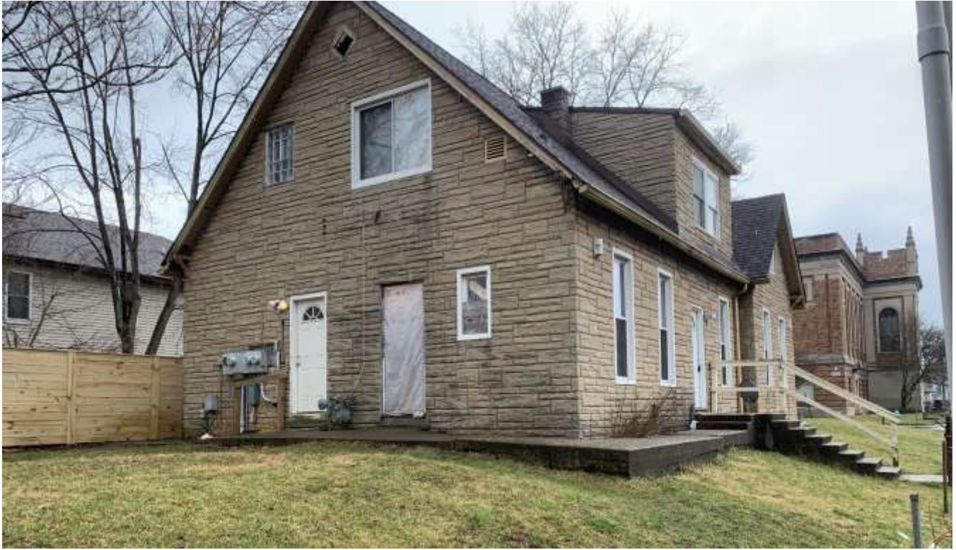
Photo of the rear building façade.
