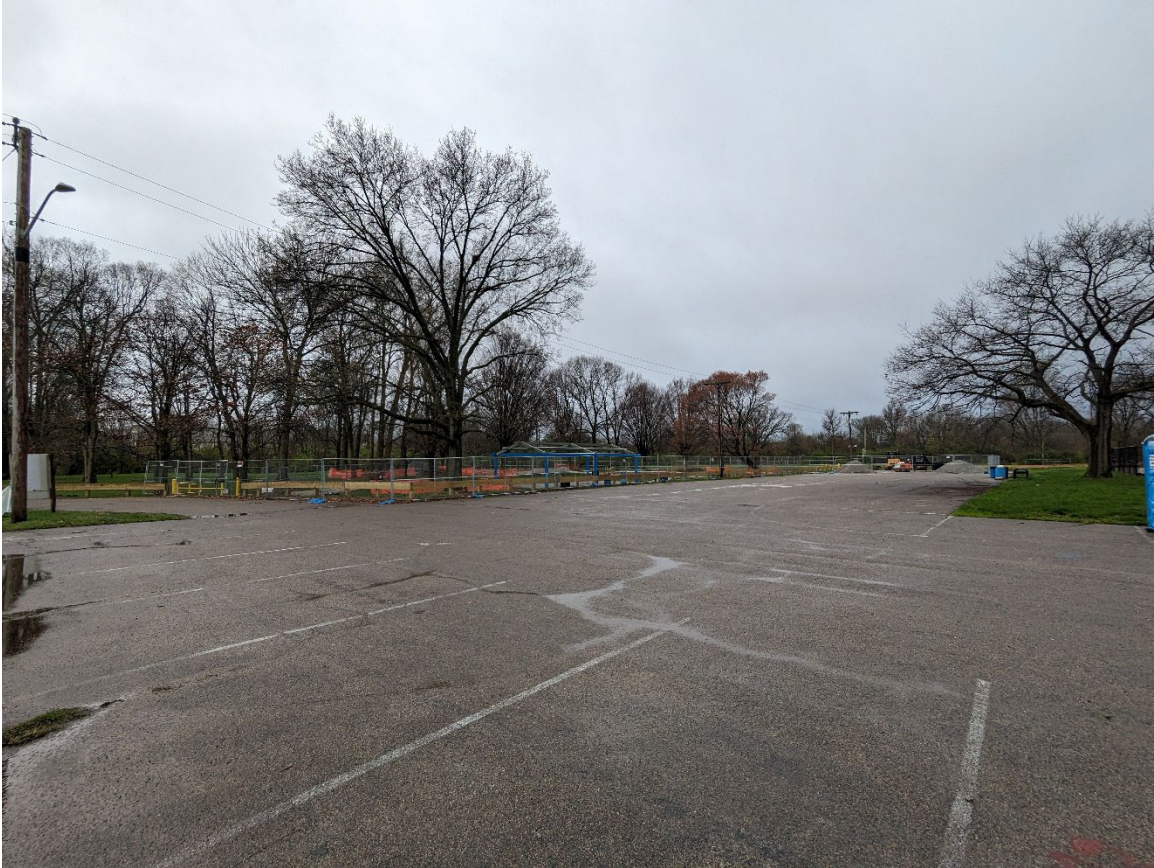
View of area of ongoing 'Playground Project' (SE area of park)
