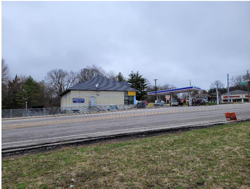
Photo 4: Adjacent Property to West of Northern Portion of Subject Site
