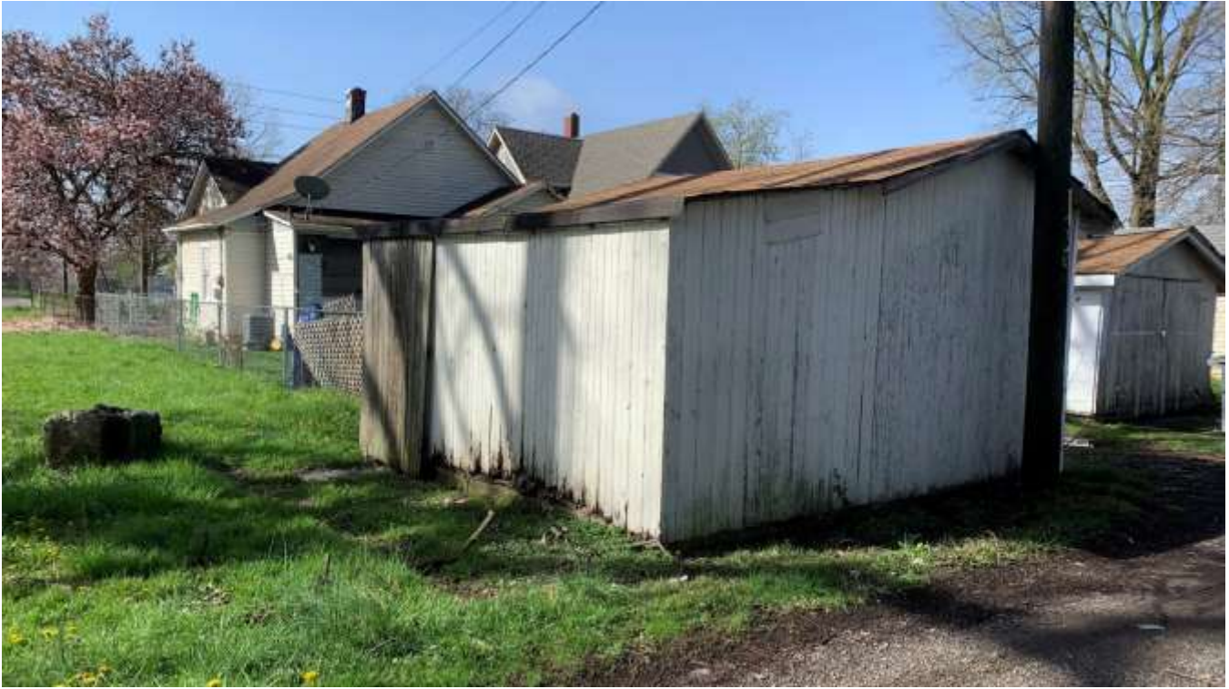
Photo of an existing shed that crosses into the subject site.
