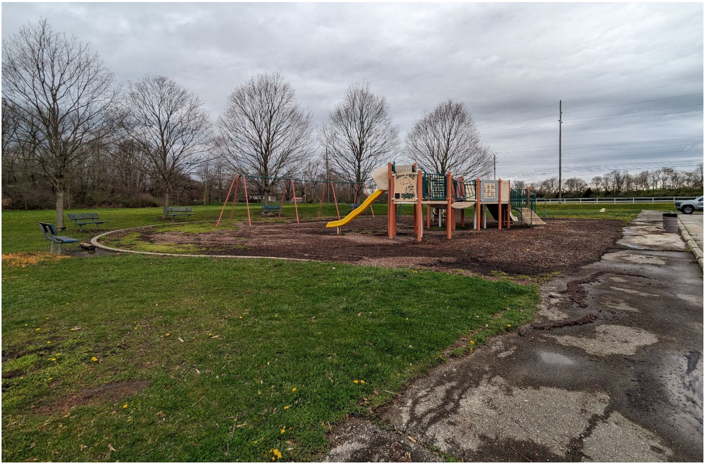
Site photo: View of existing playground
