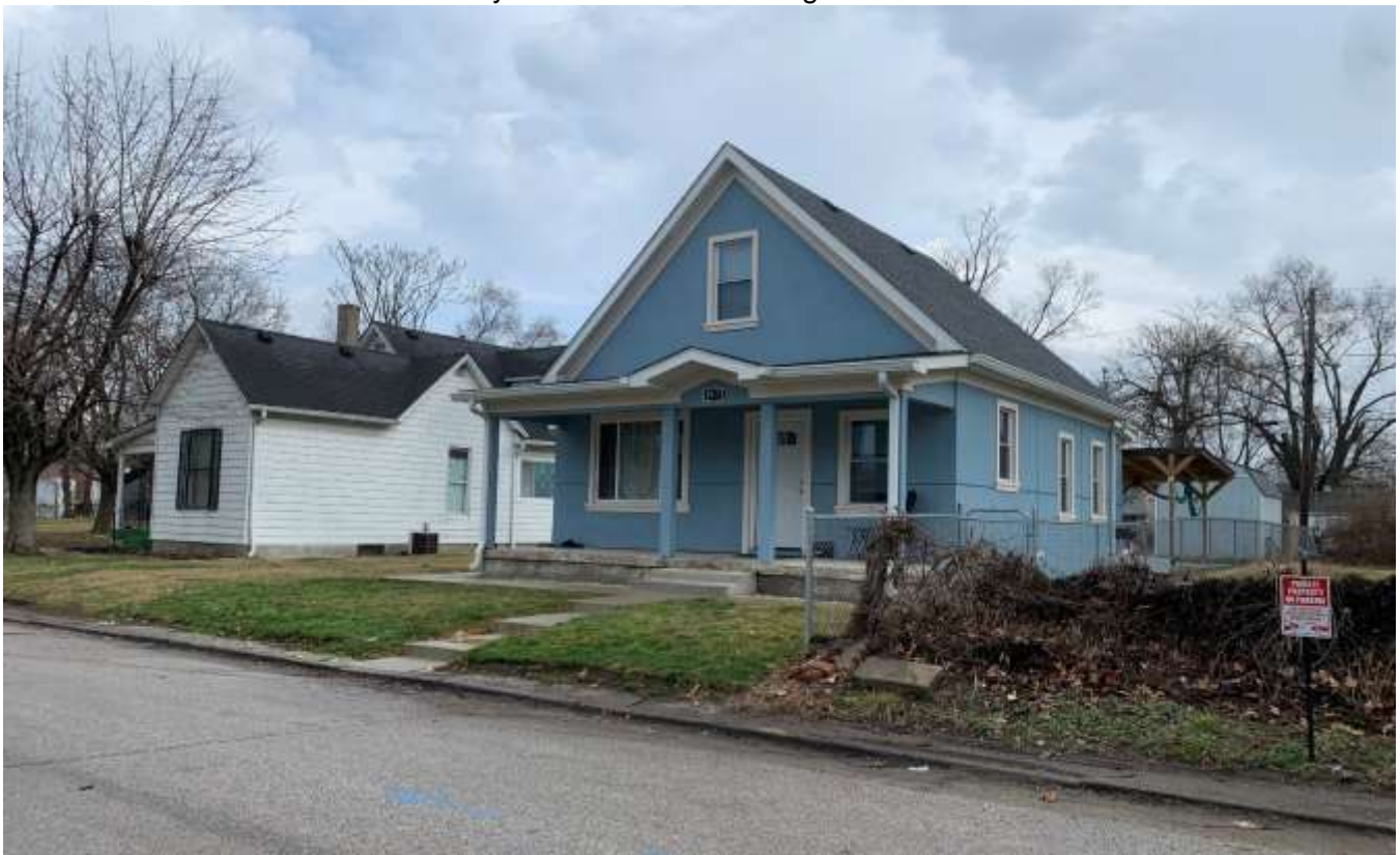
Photo of the single-family dwellings north of the site.
