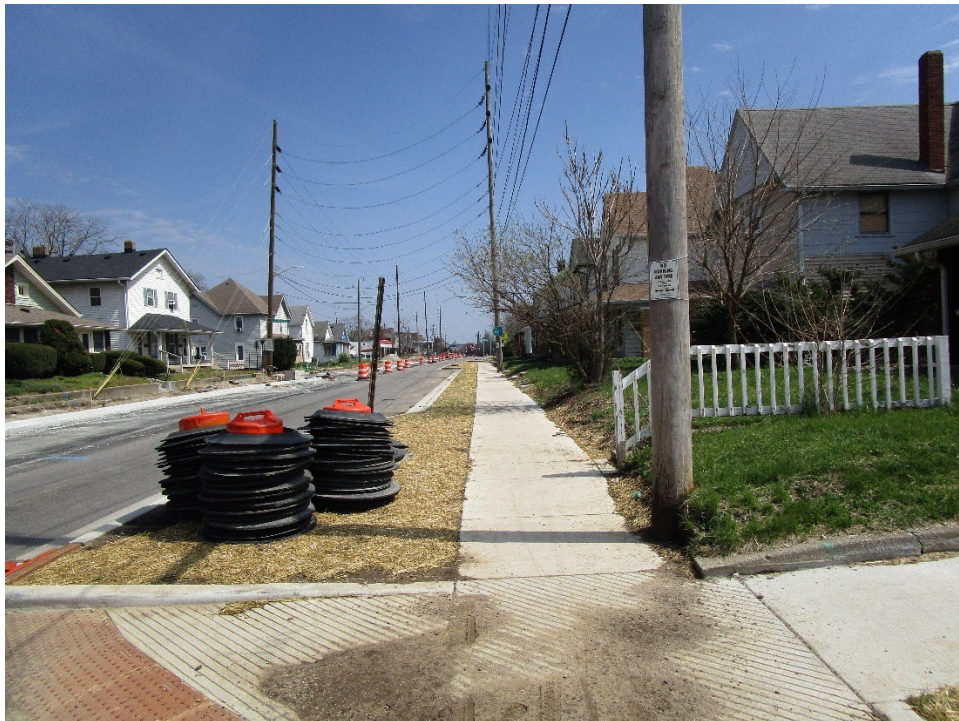
View looking east along West Morris Street
