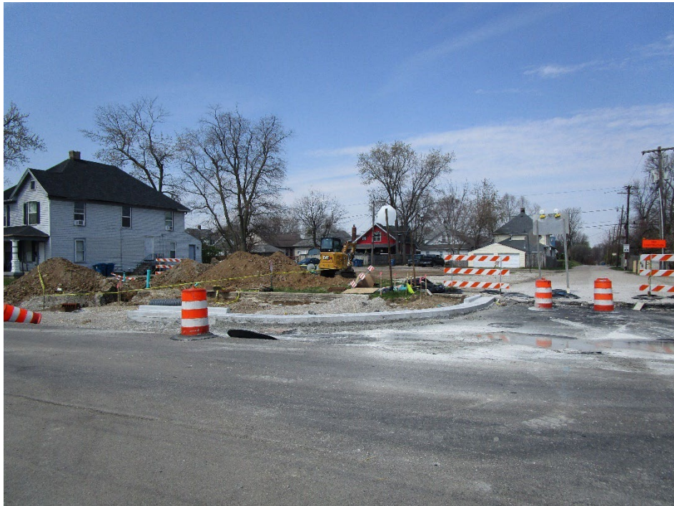
View of site looking northwest across West Morris Street / Lee Street
