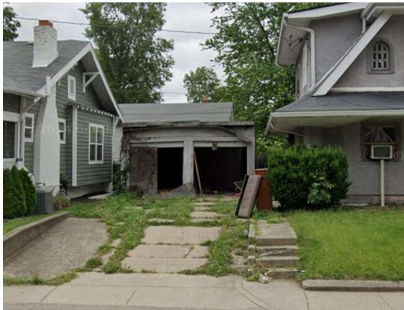
Photo 4: Previous Garage at Subject Site (June 2024)
