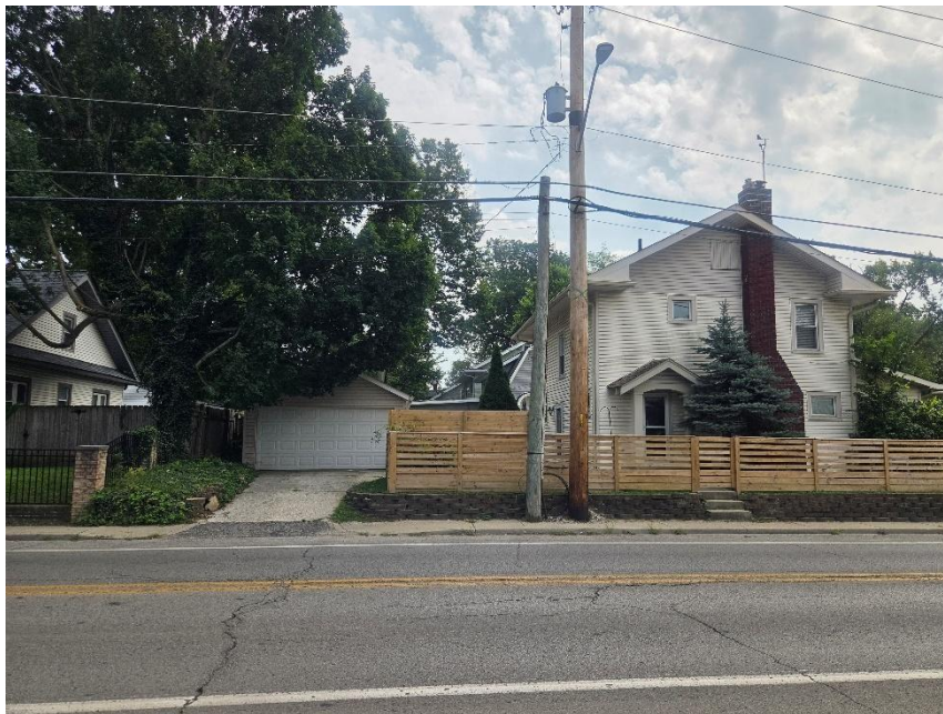
Photo 8: Non-Conforming Detached Garage at 4575 Guilford Avenue (southeast of site)
