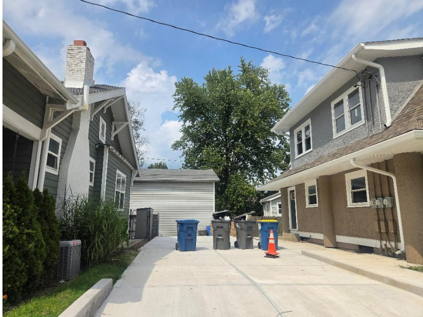
Photo 7: Proposed Garage Area Viewed from Property Line
