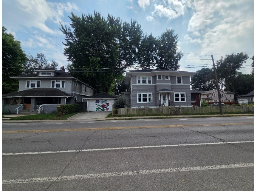
Photo 9: Non-Conforming Detached Garage at 801 E 46 th Street (southwest of site)
