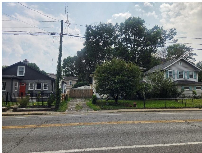
Photo 10: Non-Conforming Detached Garage at 721 E 46 th Street (southwest of site)
