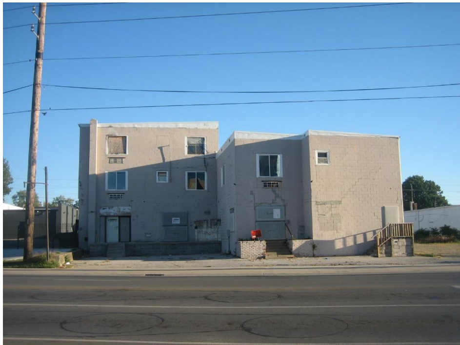
Subject site, existing building south façade, looking north from Southeastern Avenue.
