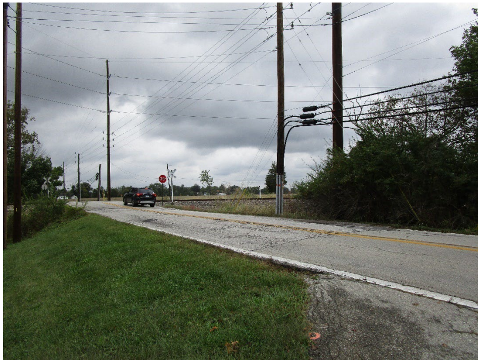
View of site looking southwest across Hickory Road
