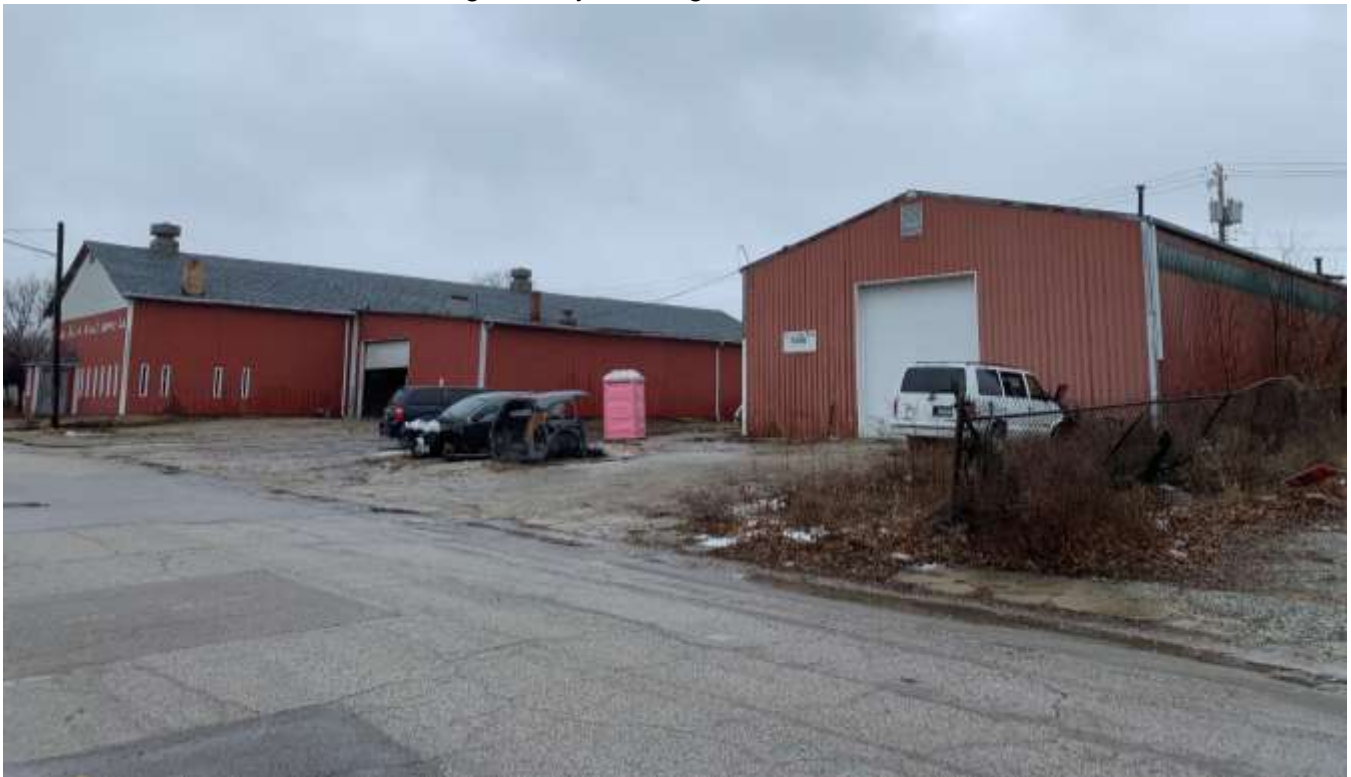
Sheet metal company north of the site.
