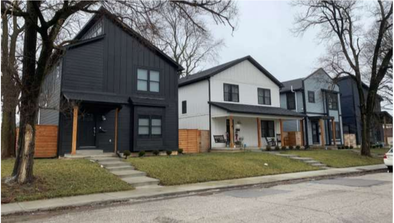
Single-family dwelling south of the site.
