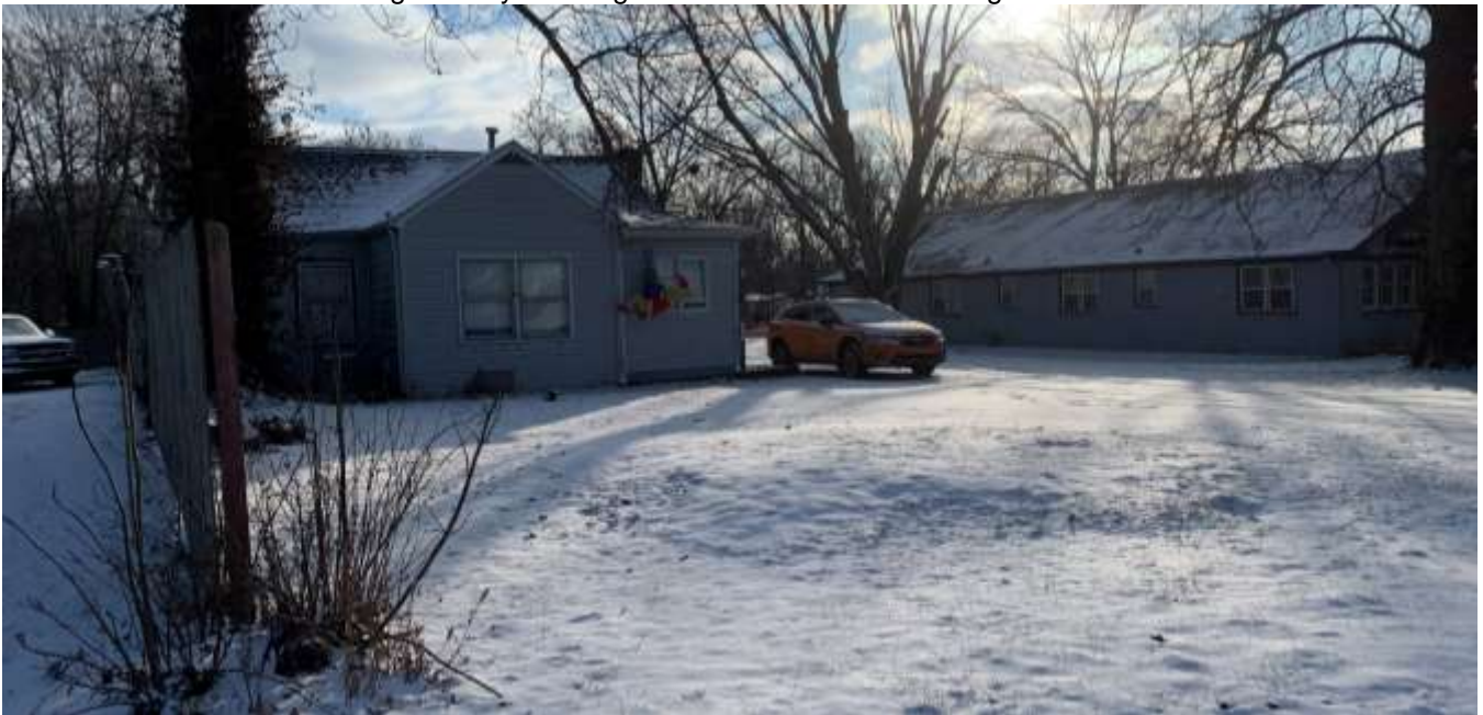
Single-family dwelling south of the site.
