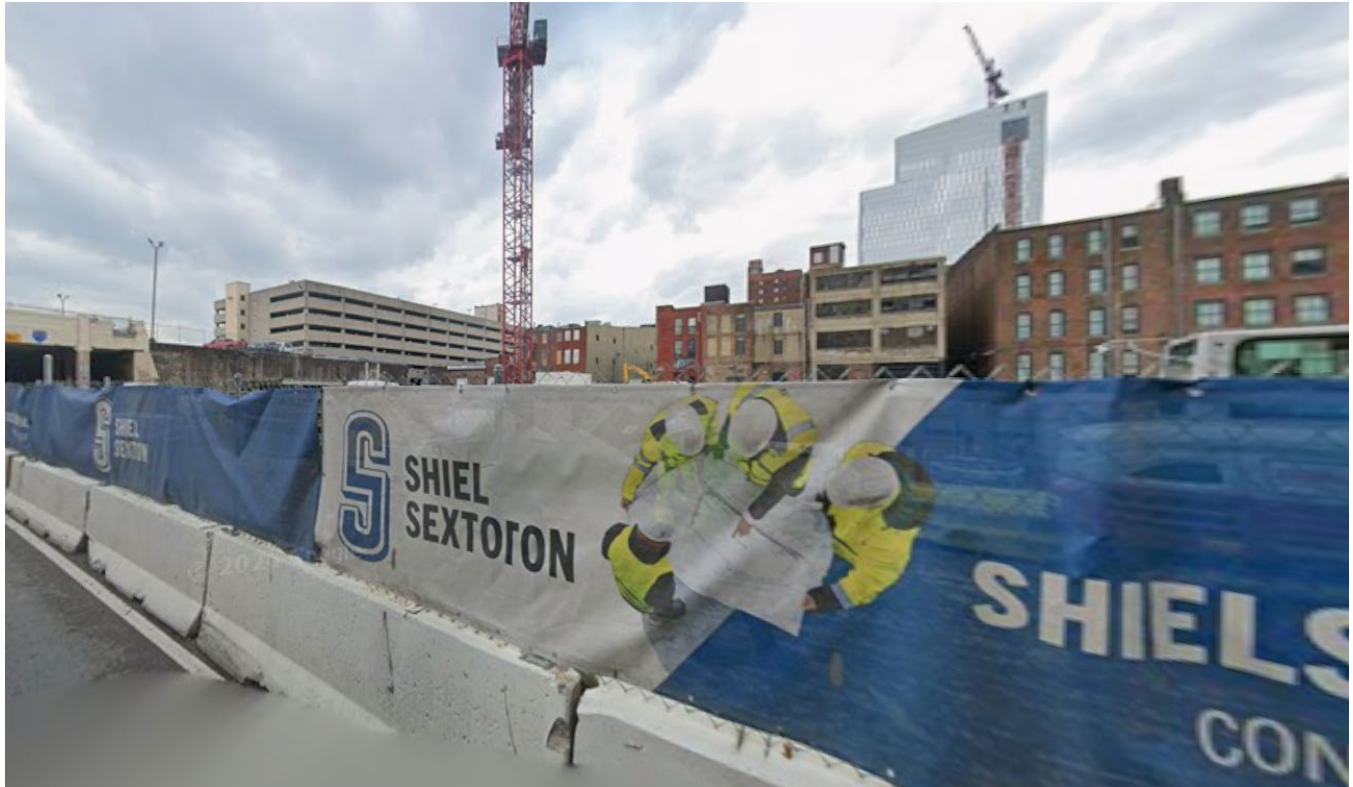
Subject Site from Pennsylvania Street (site under construction)
