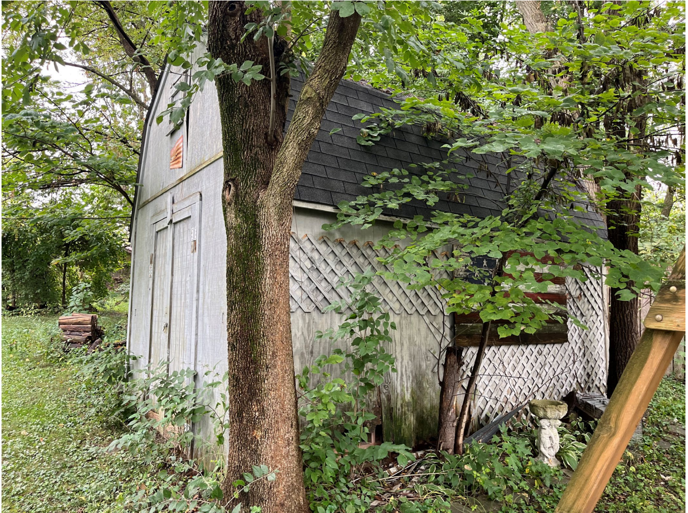
Additional view of existing shed
