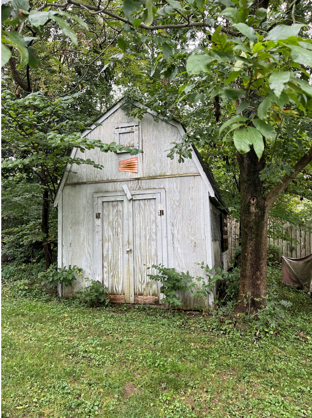
Existing shed on site
