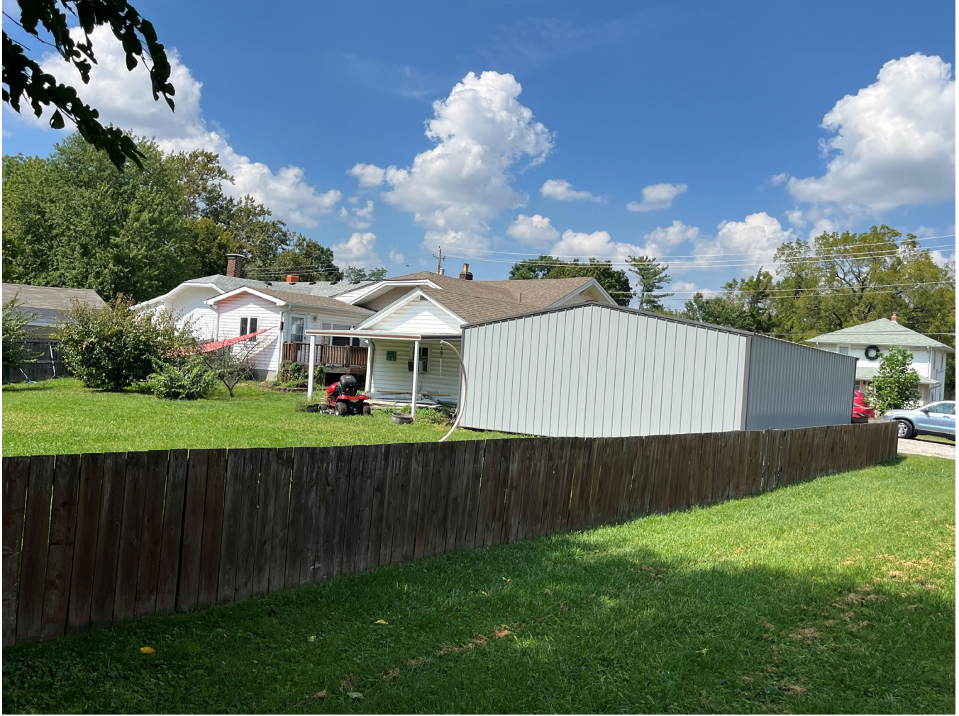
Photo 3: Partial view of backyard showing rear of both garages and house
